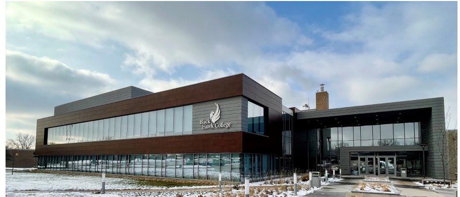
Building 1 - Addition & Renovation
