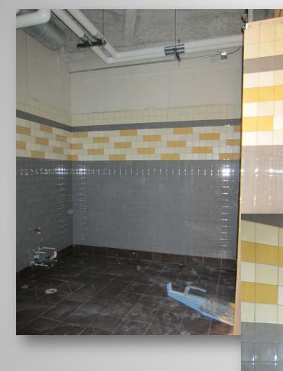
Ceramic tile has been set and grouted in bathrooms of the new addition.
